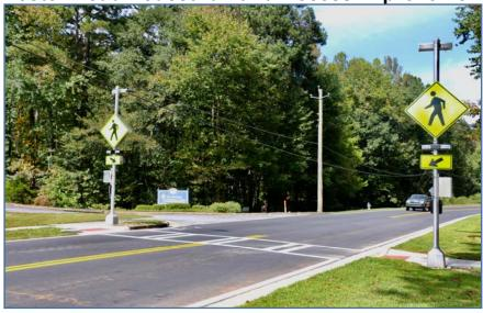
**PROJECT DESCRIPTION:** The installation 8' wide concrete sidewalk with ADA compliant wheelchair ramps, a crosswalk with rapid flashing bacons, solar panels, and push buttons, roadway resurfacing and drainage improvements
